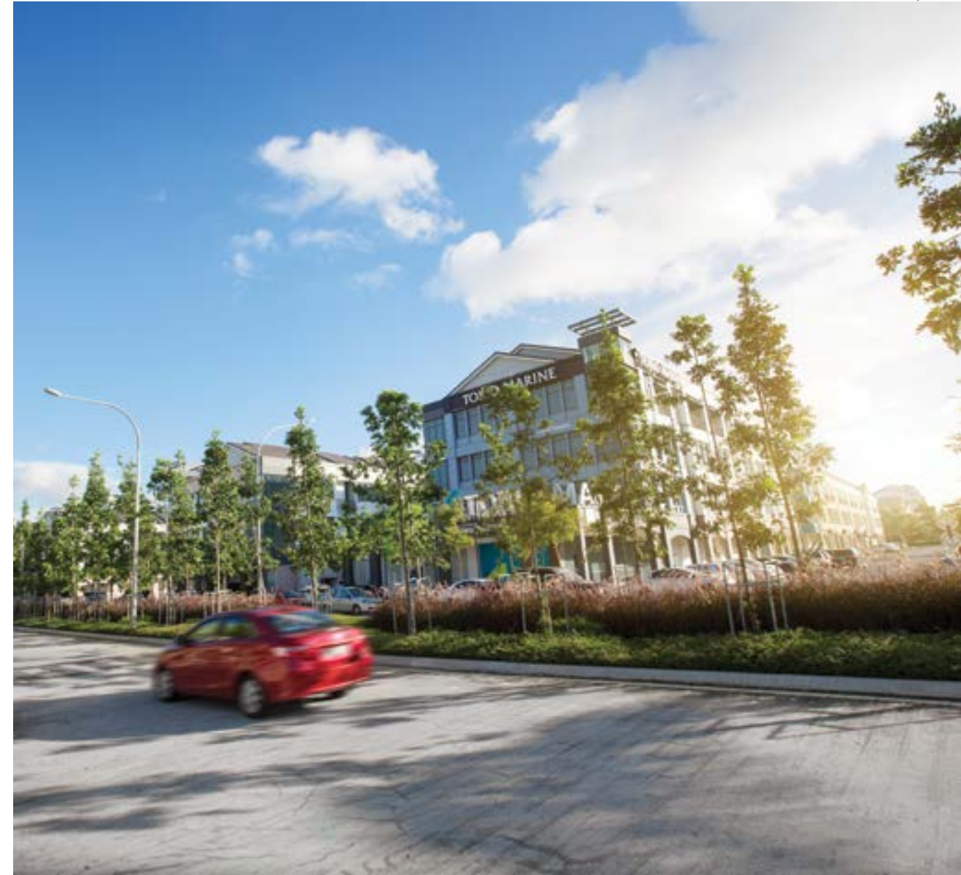
MARINA SQUARE II Completion Date : 2016
