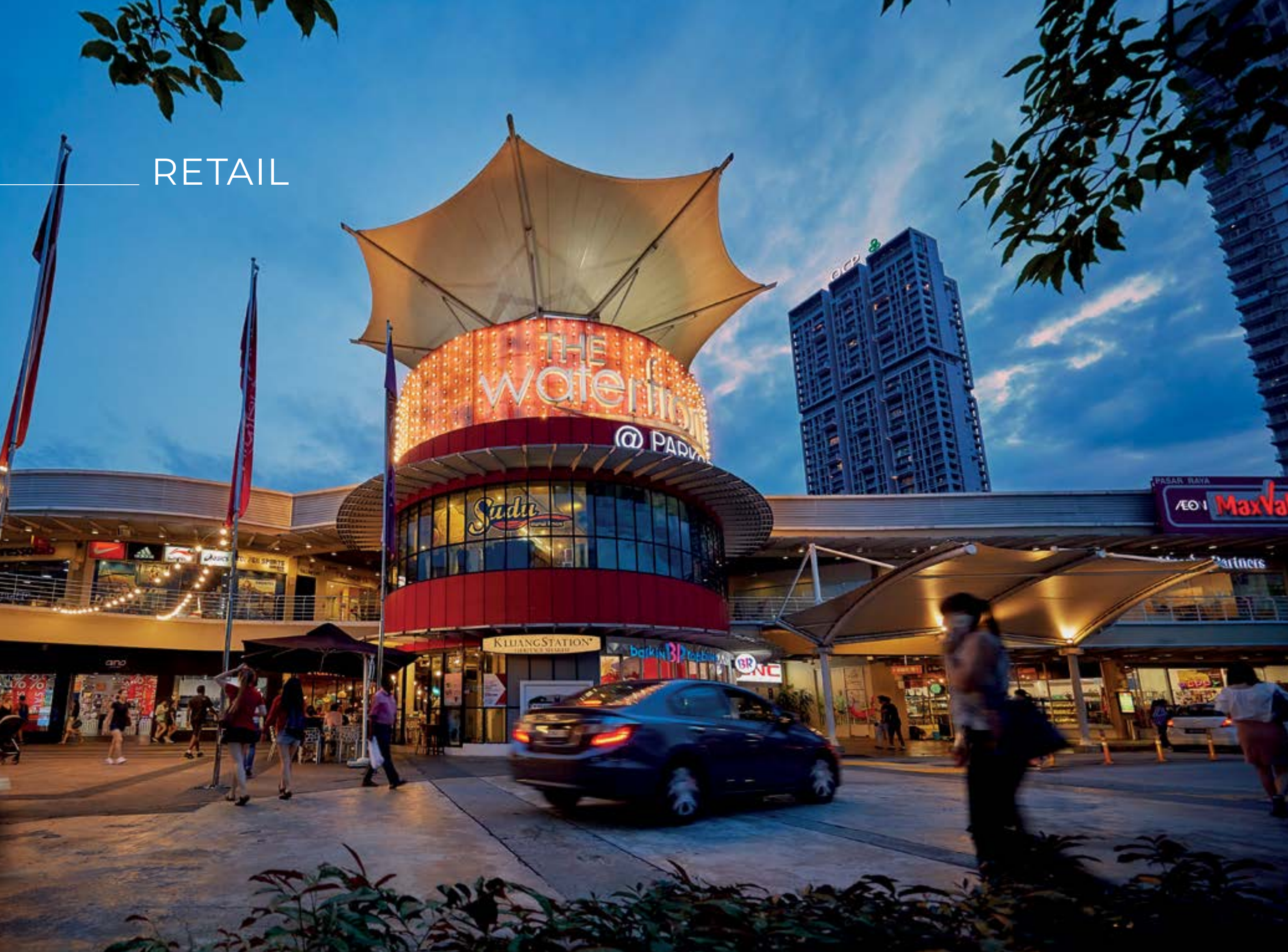
THE WATERFRONT NEIGHBOURHOOD MALL Completion Date : 2008
